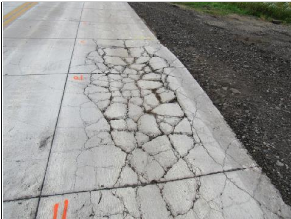
Figure 5. Shattered slabs in Cell 139.
