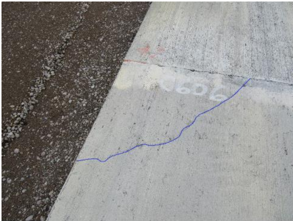
Figure 18. Corner crack in the last panel of Cell 606.
