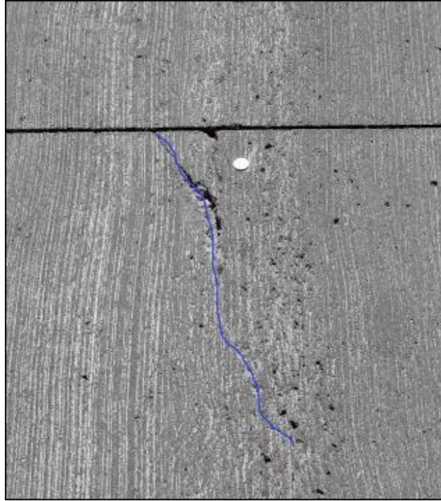
Figure 13. Longitudinal crack in Cell 805.
