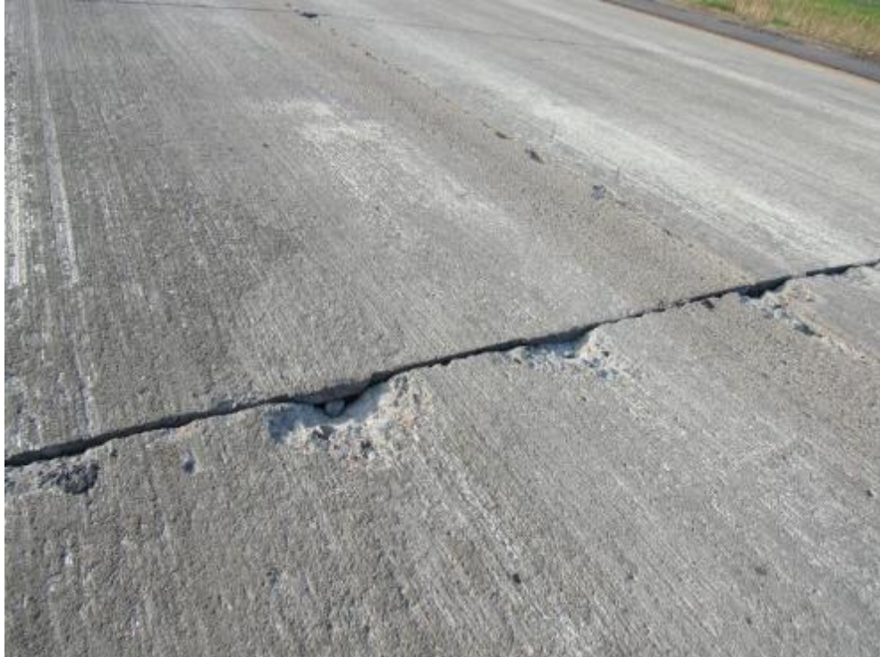
Figure 17. Spalling in Cell 506.
