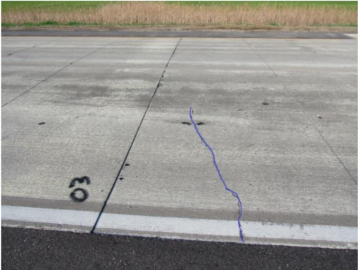
Figure 16. Transverse crack in Cell 506 (control, non-FRC).
