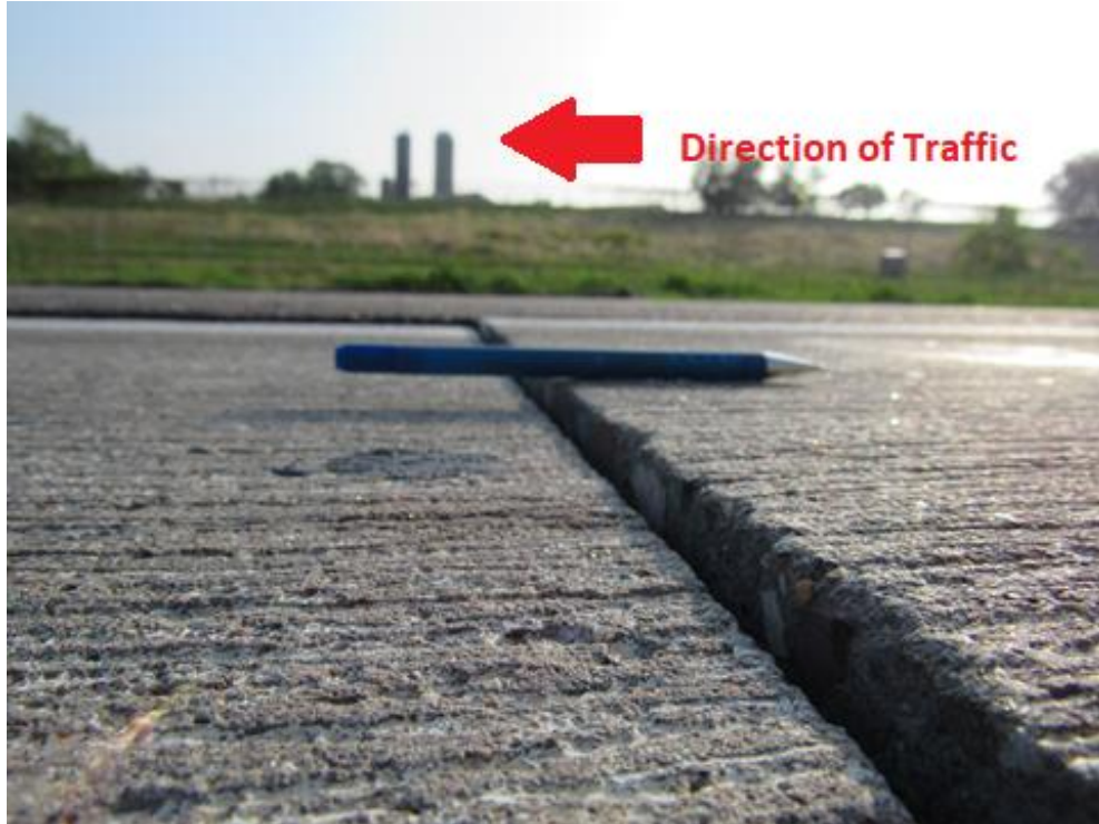
Figure 20. Photograph of faulting of Cell 506 (non-FRC). Note that faulting is exaggerated due to broken corner in slab on leave slab.
