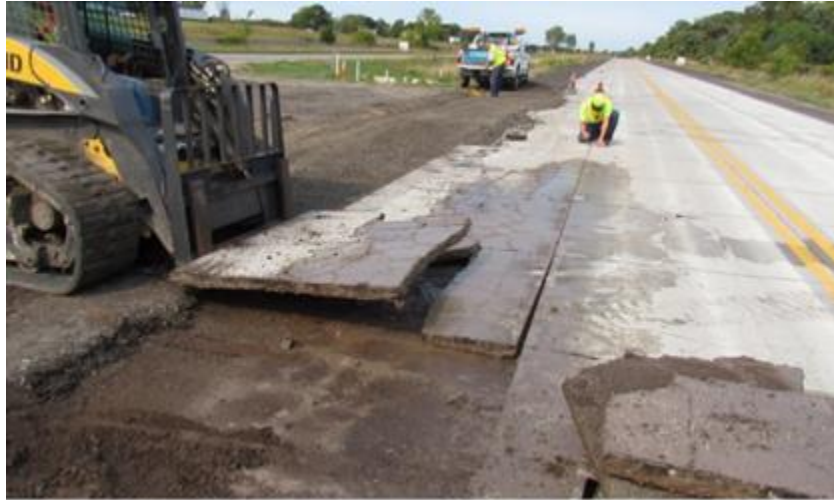
(7a) Removal of shattered slabs
