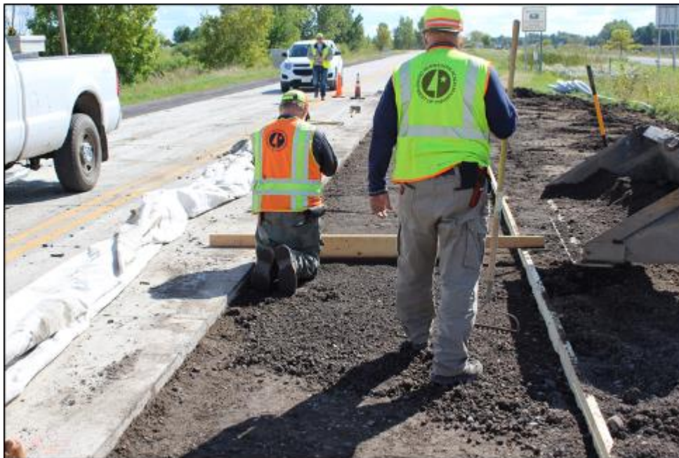
(7d) Preparation of base layer during the construction of replacement slabs.
